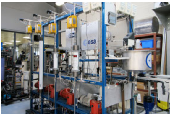
ESA PROTOTYPE – GREY WATER TREATMENT UNIT
